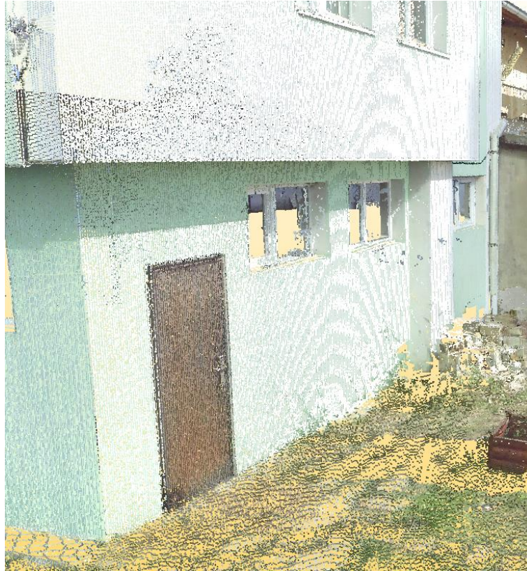
Fig. 1 3D laser scanning of administrative building with various shapes
