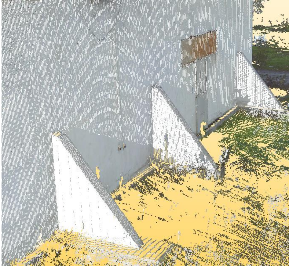
Fig. 2 3D laser scanning of specific cadastral details of an industrial building
